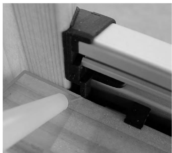
Integrally moulded sealing compound channels facilitate the sealing of the end cap to the timber blind frame.
